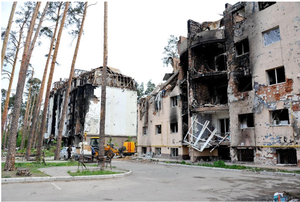
Figure 2: Demolition works in the city of Irpin
